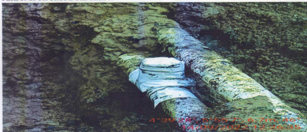
PICTURE 1: SHOWING 3" FLANGE INSTALLED AT THE INCIDENT POINT BY UNKNOWN PERSONS FOR CRUDE OIL THEFT.
