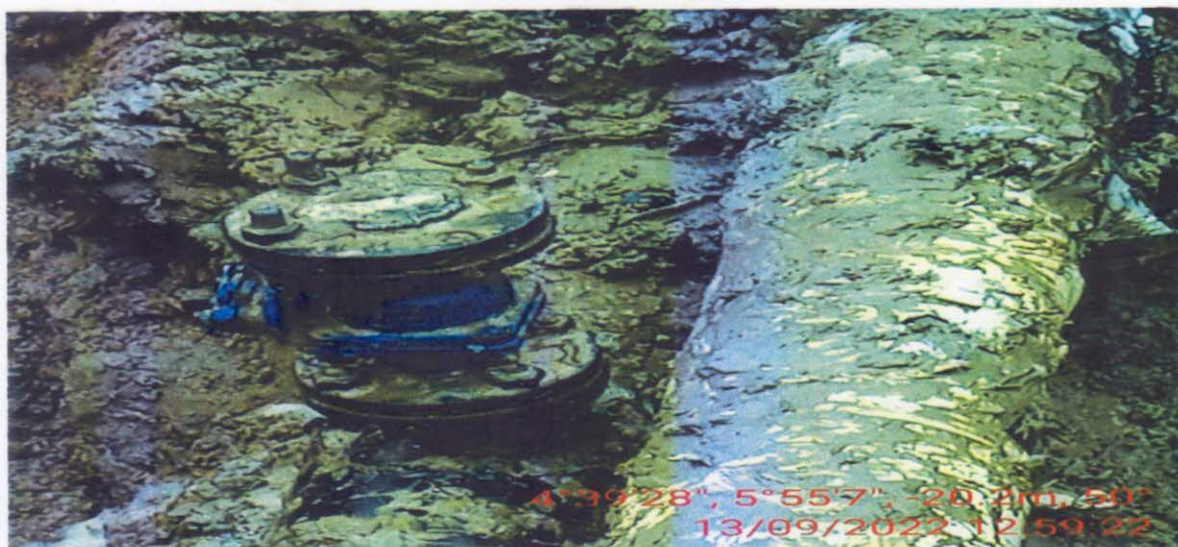
PICTURE 1: SHOWING 3" FLANGE INSTALLED AT THE INCIDENT POINT BY UNKNOWN PERSONS FOR CRUDE OIL THEFT.
